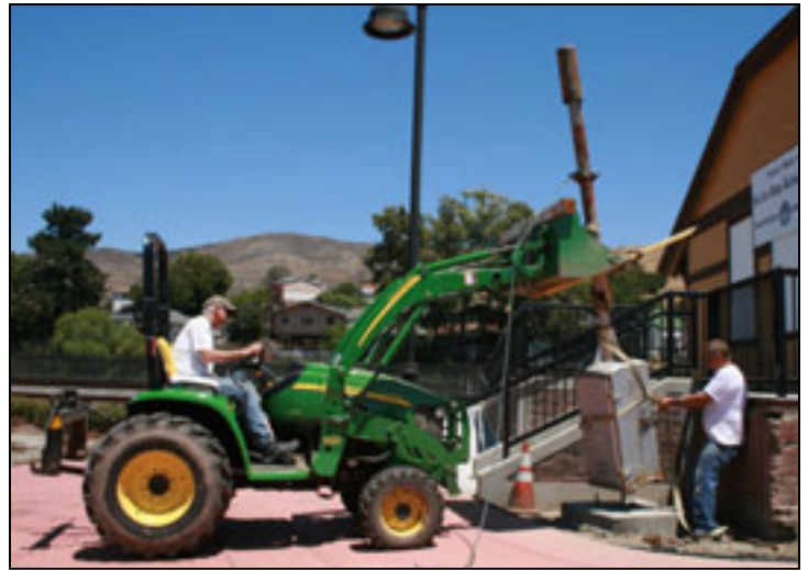
Howard Amborn uses his trusty tractor to lift the Wig-Wag while Ted VanKlaveren wrestles it into place. This antique crossing signal will be used to indicate when the Museum is open to the public. Photo by Gary See
