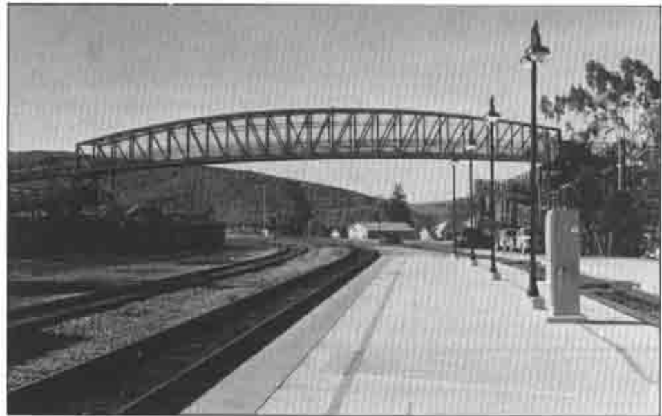
Jennifer Street footbridge
