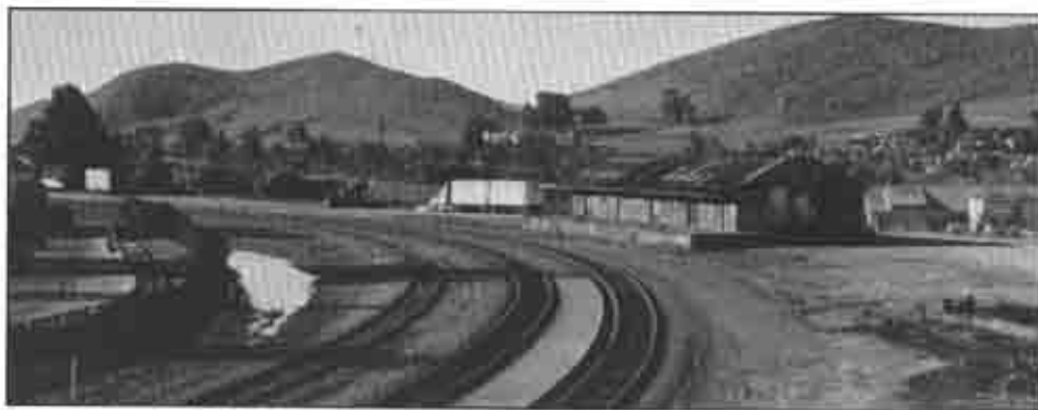
1893 Southern Pacific Freight Warehouse viewed from the Jennifer Street Bridge.
