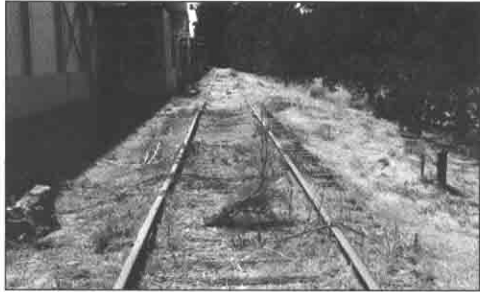
Spur track along the side of the Atoll Business Park south building.
