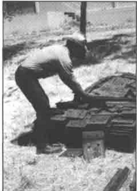
Brad LaRose stacking tie-plates.
