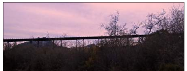
Stenner Canyon Trestle in Fall 2015.
