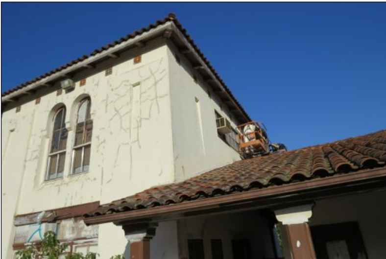
Above, a bucket truck allows a worker to safely prepare the depot's second story. Below, a crew from Ellison's Painting of Merced puts finishing touches on the former Railway Express Agency building, which needed stucco repair. Including the bus shelter and REA building allowed economies of scale.
