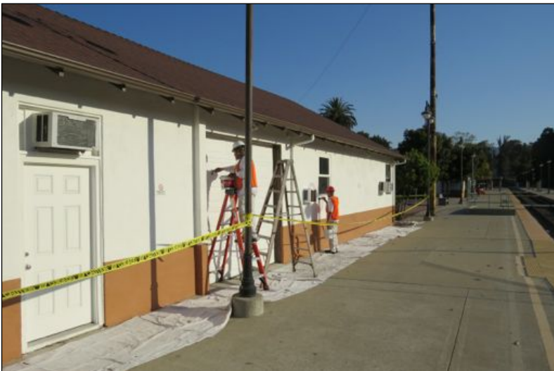
Above, a bucket truck allows a worker to safely prepare the depot's second story. Below, a crew from Ellison's Painting of Merced puts finishing touches on the former Railway Express Agency building, which needed stucco repair. Including the bus shelter and REA building allowed economies of scale.
