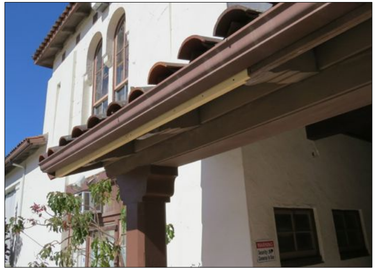
Above, we see attention to detail for replacement wood trim, not yet painted, carefully lap-jointed and (not visible in this view) mitered at the outer corner.
