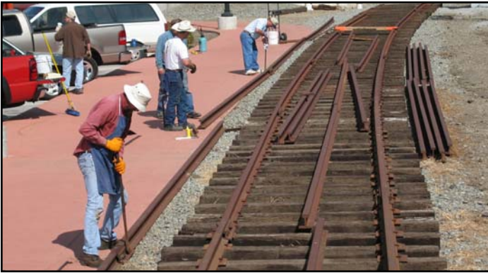
Bill Rust and Karl Hovanitz tighten track bolts while Brad LaRose and Ted VanKlavern plot their next move.
