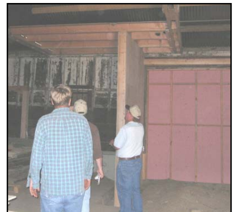
Ted VanKlavern, Aron Kahn and Karl Hovanitz inspect the shear walls.
