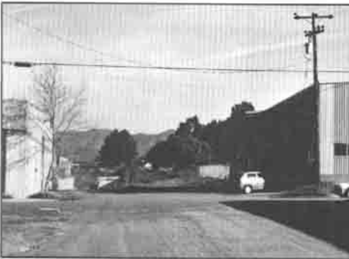
Emily Street, looking north. Sears warehouse is on right.
