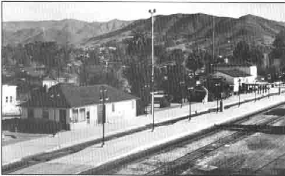
REA Building is on right, looking northeast from Jennifer Street Bridge.
