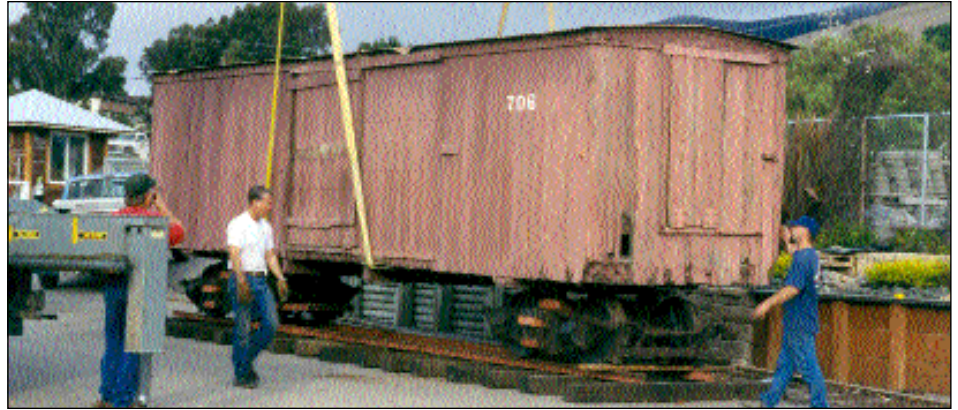
Pacific Coast Railway boxcar #706 is gently lowered onto the Westside Lumber Company narrow gauge trucks at the Pacific Home and Garden Center yard.
