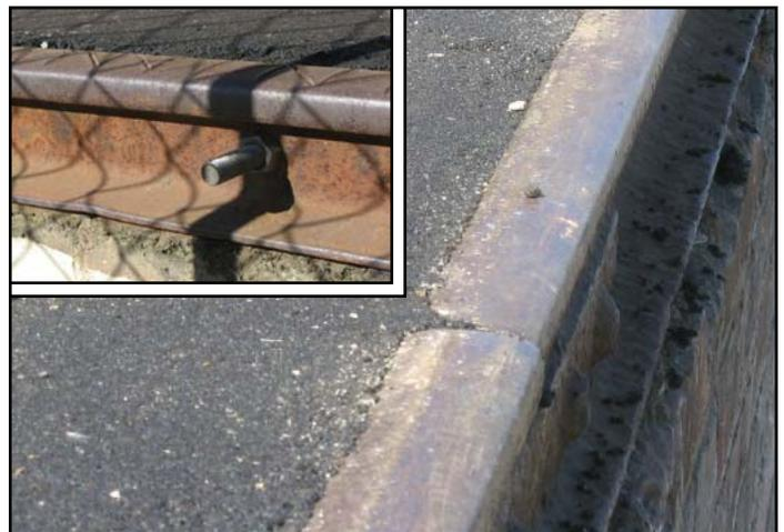
Old rail used as edging for the trackside platform has been bolted in place and holes in the asphalt filled in.
