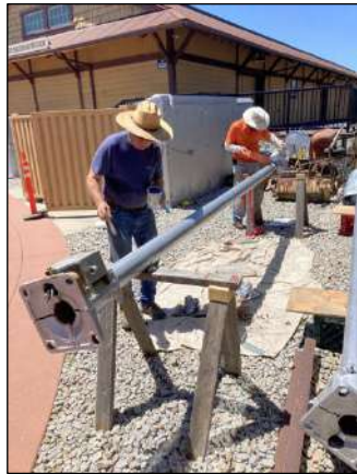
Before signals were installed they were cleaned and painted (above left). With the pandemic a memory, tours by school groups resumed (below).
